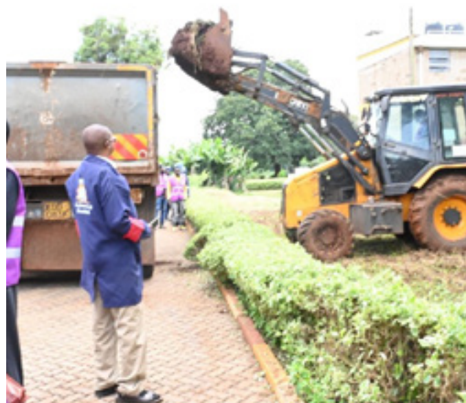
Contractors at the site.
